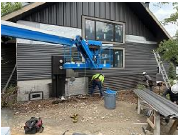
Building C10 Unit 70 Side Corrugated & Lap Siding Installed
