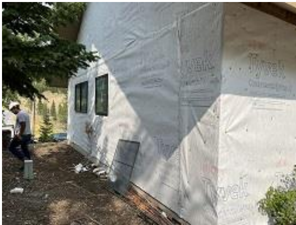
Building B Unit 7 Side Windows Installed
