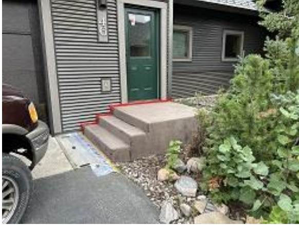
Building E6 Unit 46 Stoop Refinishing Continued
