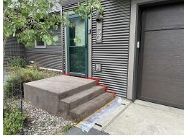
Building E7 Unit 50 Stoop Refinishing Began
