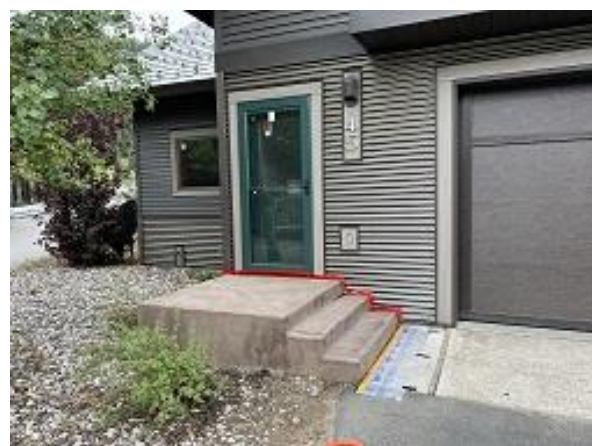
Building E6 Unit 45 Stoop Refinishing Continued
