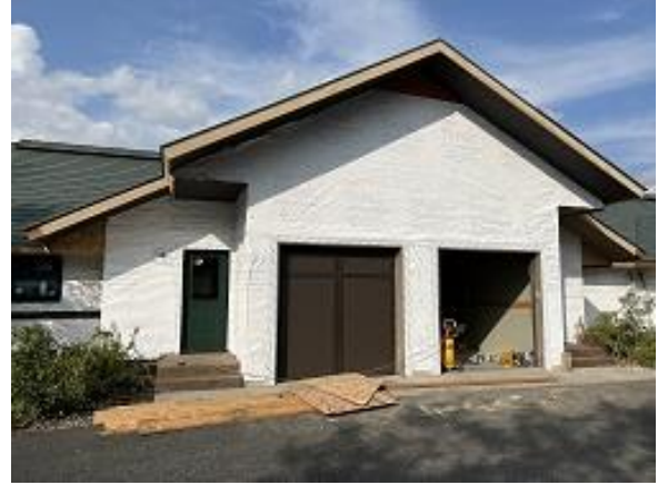
Building B Units 6 & 7 Front Soffit Installed
