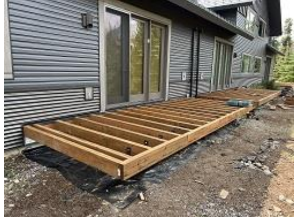
Building E8 Units 56 & 57 Deck Framing
