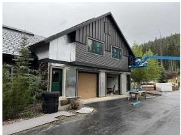
Building C10 Units 69 & 70 Front Lap Siding Installed
