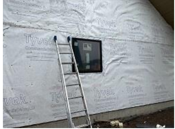
Building B Unit 3 Side Window Installed
