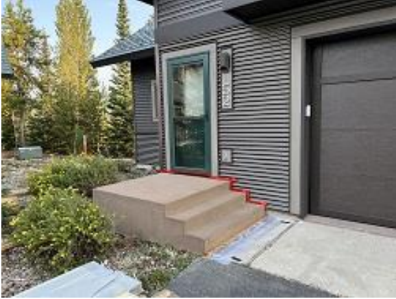
Building E7 Unit 58 Stoop Concrete Coating Applied
