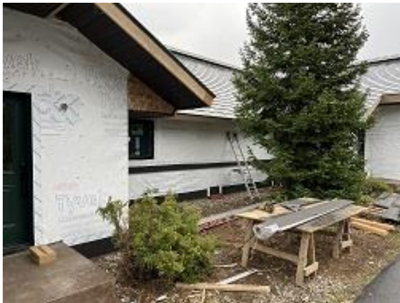
Building B Units 4 & 5 Front Base & Wainscot Flashing Installed
