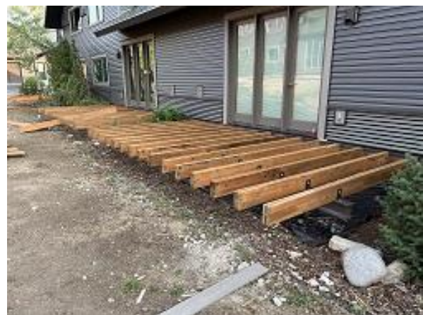
Building E6 Units 46 - 48 Deck Framing
