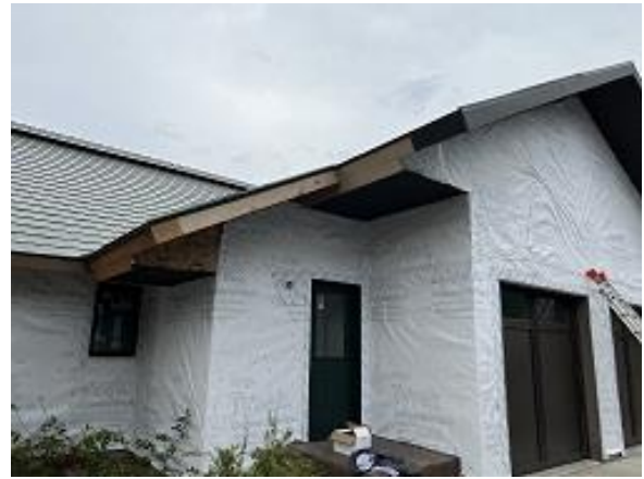
Building B Unit 4 Soffit & Fascia Installed
