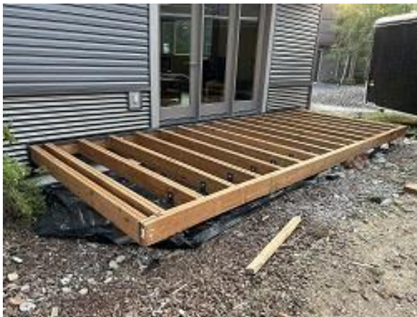
Building E6 Unit 45 Deck Framed
