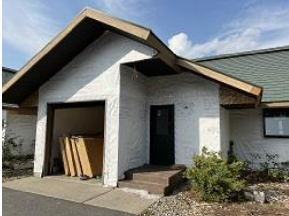
Building B Units 5 Front Soffit Installed
