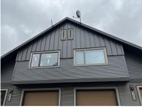
Building C9 Units 67 & 68 Satellite Dishes Installed
