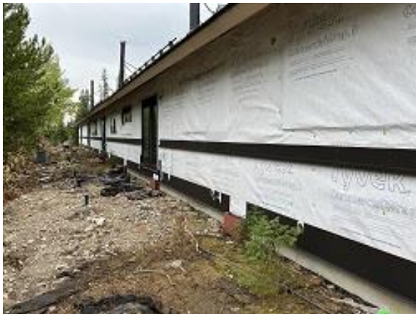
Building B Units 3 - 7 Back Base & Wainscot Flashing Installed
