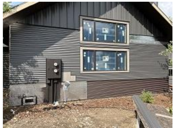
Building C10 Units 70 Side Lap Siding Installed
