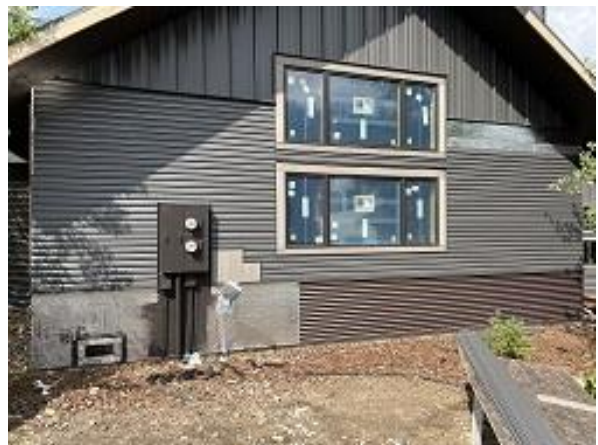
Building C10 Units 70 Side Lap Siding Installed
