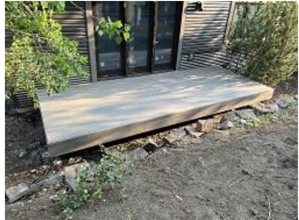
Building C2 Unit 15 Decking Installed
