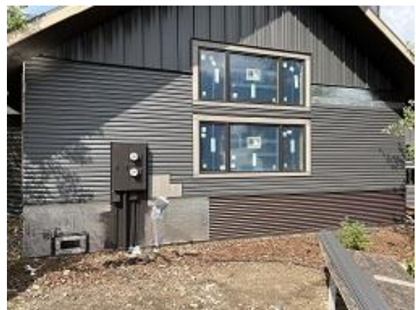
Building C10 Units 70 Side Lap Siding Installed
