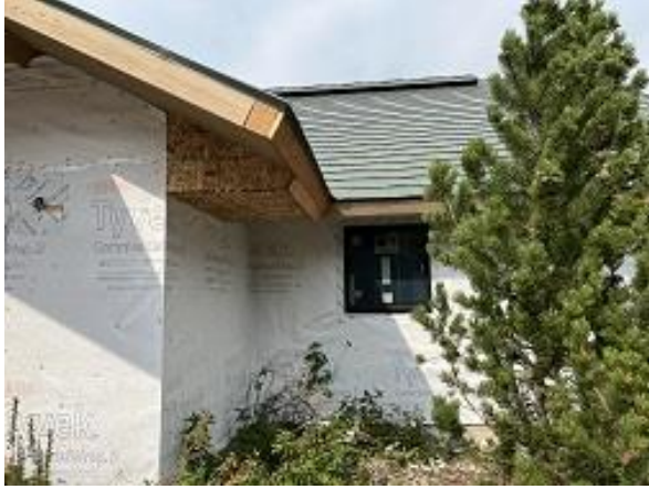
Building B Unit 3 Kitchen Window Installed & Rafter Repair Completed
