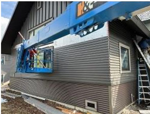
Building C10 Units 69 Side & Front Lap Siding Installed
