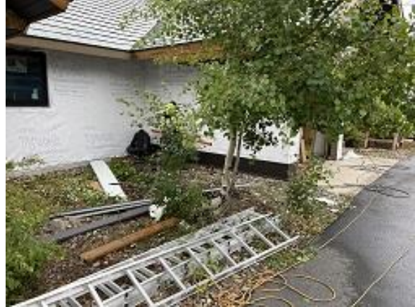
Building B Unit 5 Front Base Flashing Installed
