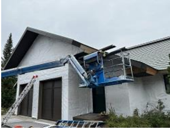
Building B Unit 3 Soffit & Fascia Installed
