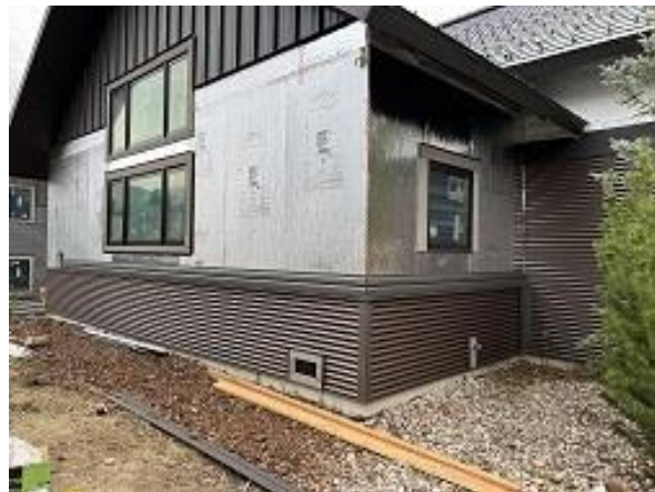
Building C10 Unit 69 Front & Side Corrugated Siding Installed
