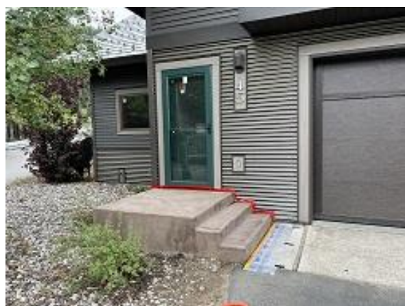
Building E6 Unit 45 Stoop Refinishing Continued
