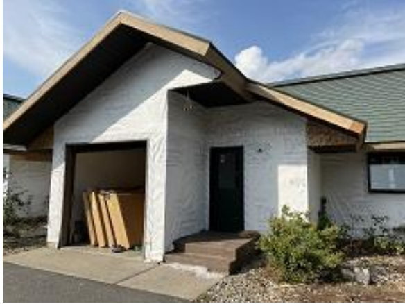
Building B Units 5 Front Soffit Installed
