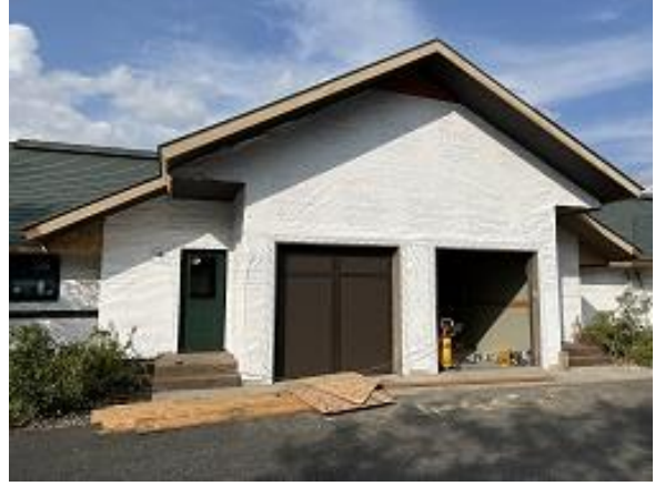
Building B Units 6 & 7 Front Soffit Installed
