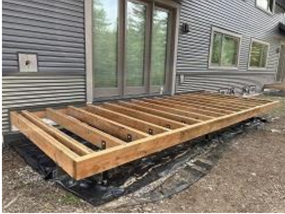
Building E8 Unit 55 Deck Framing
