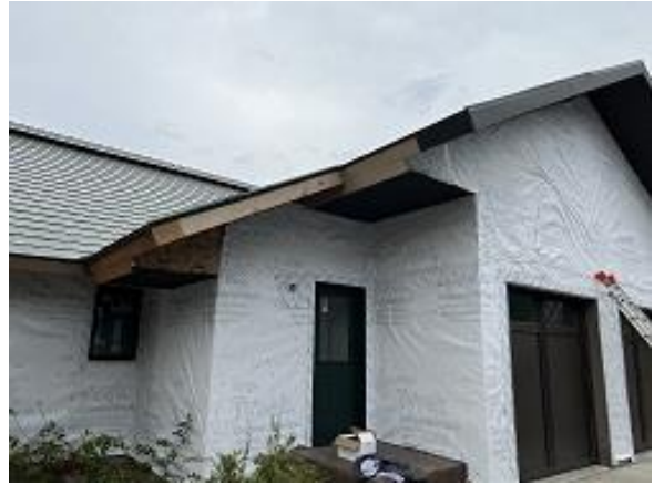
Building B Unit 4 Soffit & Fascia Installed
