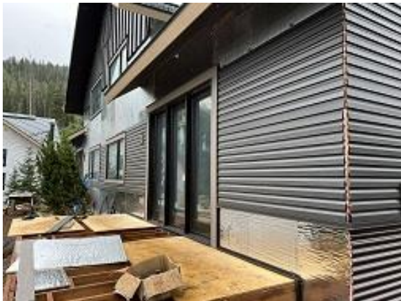
Building C10 Units 69 & 70 Back Lap Siding Installed
