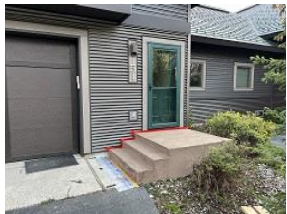
Building E7 Unit 51 Stoop Concrete Coating Applied
