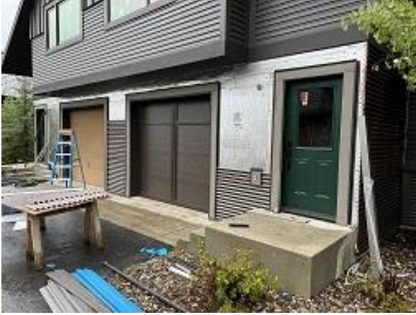
Building C10 Units 69 & 70 Front Corrugated Siding Installed
