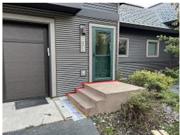
Building E7 Unit 51 Stoop Concrete Coating Applied
