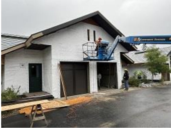
Building B Units 6 & 7 Front Louvers Cut In
