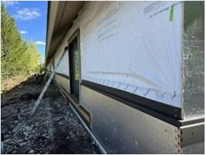
Building B Unit 7 Back Foam Board & Door Trim Installed
