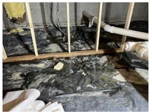
Building E5 Unit 43 Crawl Space Standing Water At Sump Pump
