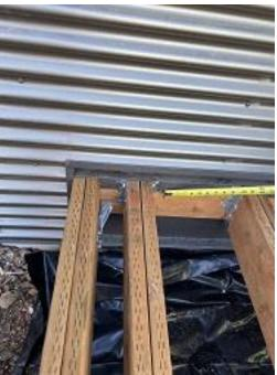
Building E9 Unit 61 Observed Incorrect Joist Hanger Installed
