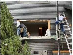
Unit 60 Back Lower Window Install Removing Insulation Board behind Siding & Cut Tyvek
