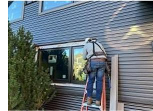
Building C7 Unit 60 Back Lower Window Observed Tyvek Cut At J Channel
