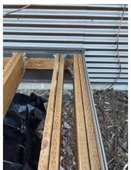
Building E9 Unit 62 Observed Incorrect Deck Joist Hanger Installed
