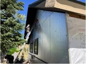
Building B Unit 7 Side Foam Board, J Channel, Trim Installed
