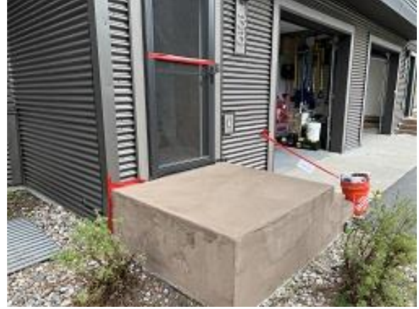
Building C3 Unit 33 Stoop Coating Began
