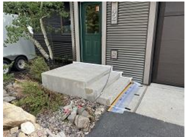
Building E5 Unit 42 Stoop Coating Began
