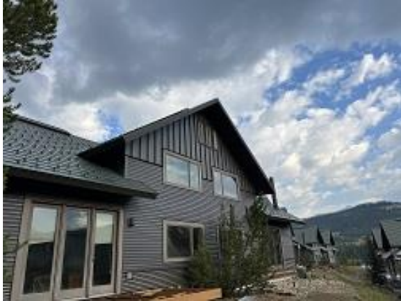
Building C3 Unit 33 Back Bathroom Vents Blockout Installed
