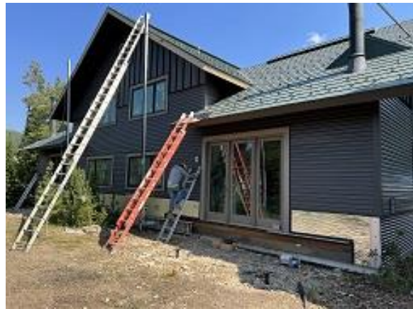
Building C6 Units 53 & 54 Back Snap Batten & Lap Siding Installed
