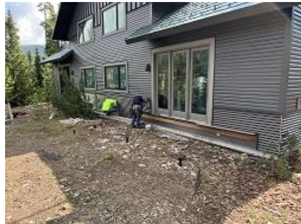
Building C6 Units 53 & 54 Back Corrugated Siding Installed
