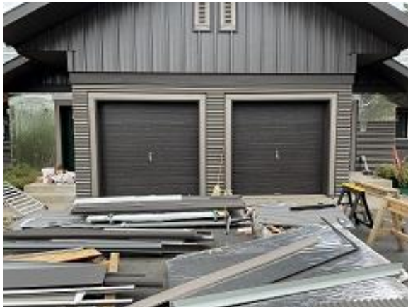
Building A Units 1 & 2 Front Corrugated Siding Installed
