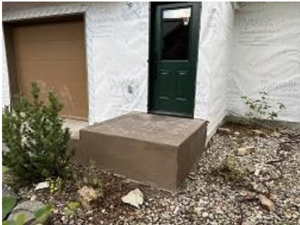
Building C4 Unit 35 Stoop Coating Began
