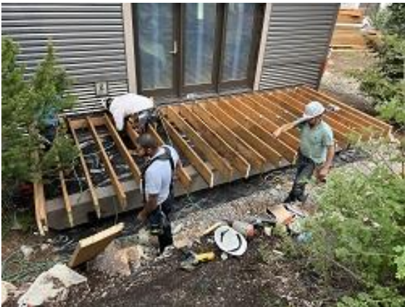
Building C2 Unit 14 Deck Framing
