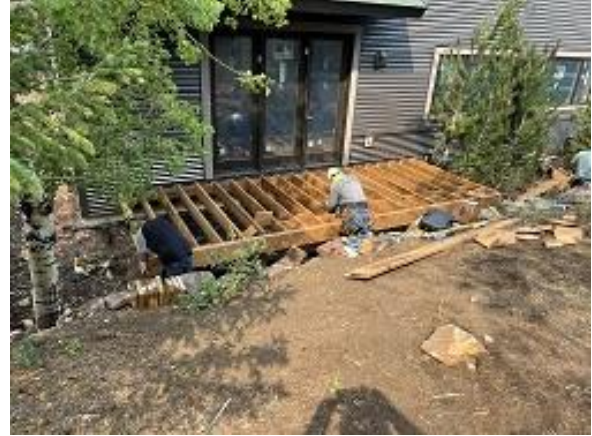
Building C2 Unit 15 Deck Framing
