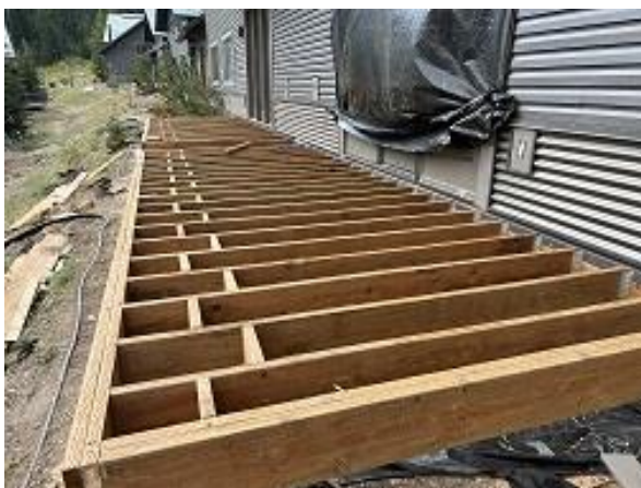
Building E5 Unit 43 Deck Framing
