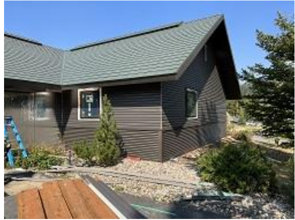
Building A Unit 1 Kitchen & Side Windows Reinstalled
