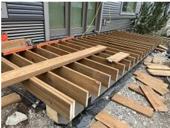
Building E5 Unit 41 Deck Framing Began
