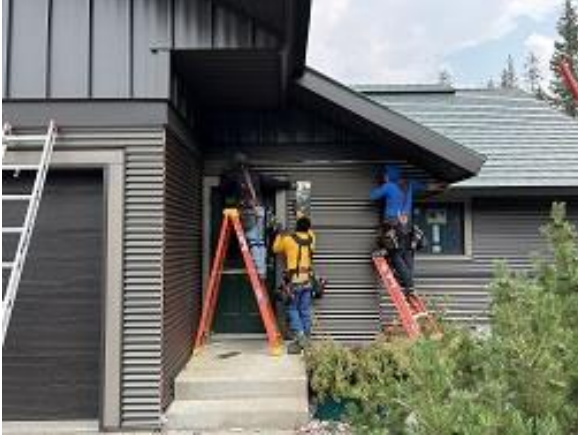
Building A Unit 1 Front Corrugated Siding Installed
