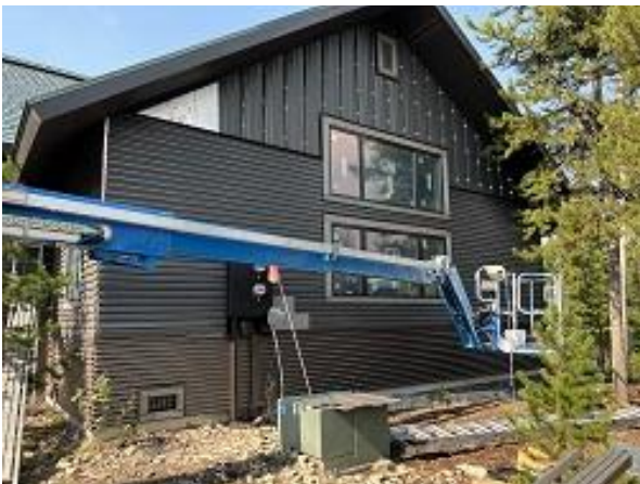
Building C6 Unit 53 Side Snap Batten Siding Installed
