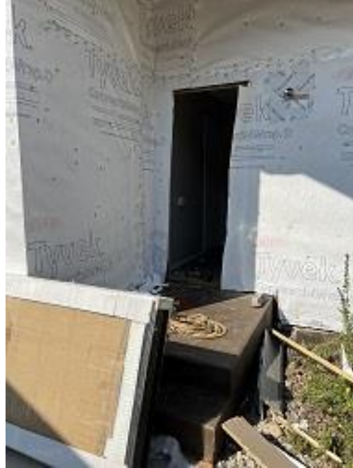
Building B Unit 3 Front Door Removed
