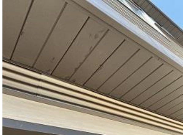
Building C6 Unit 53 Front Soffit Touch Up Paint
