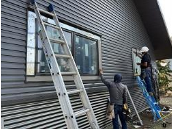
Building A Unit 2 Side Windows Trim Reinstalled
