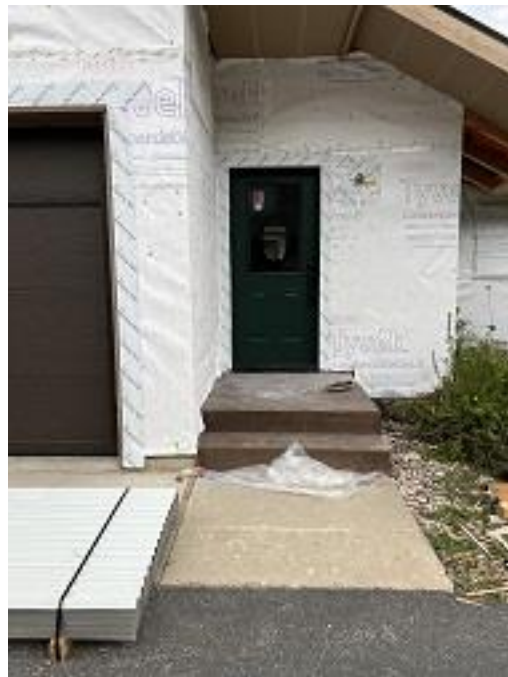
Building B Unit 3 Front Door Installed
