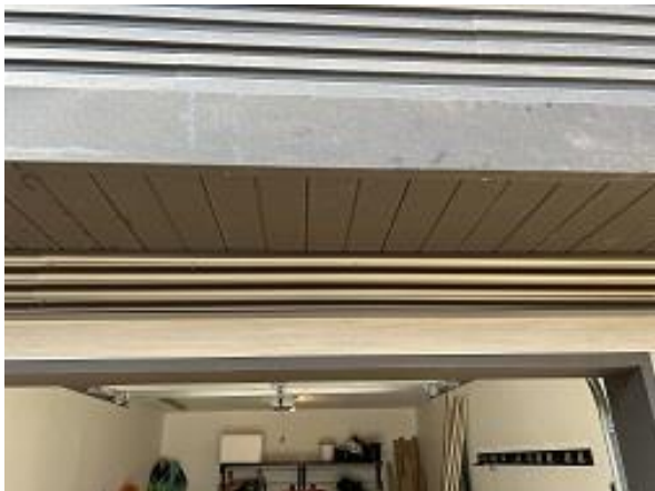
Building C6 Unit 53 Front Belly Band Touch Up Paint
