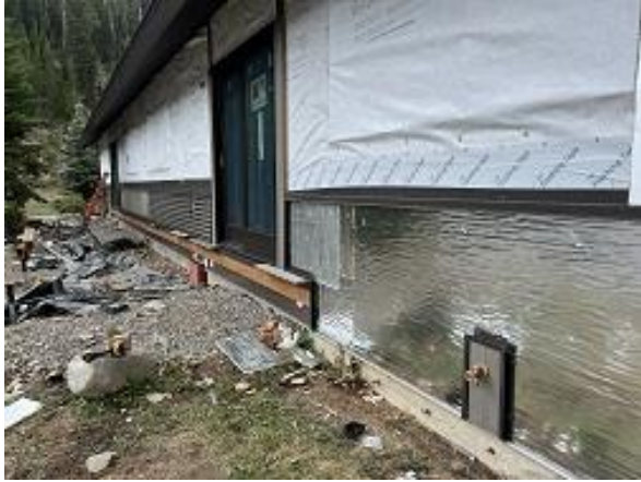
Building A Units 1 & 2 Back Corrugated Siding Installed
