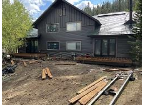
Building C1 Units 12 & 13 Deck Framing
