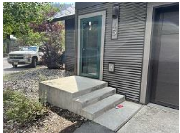
Building E6 Unit 45 Stoop Coating Began
