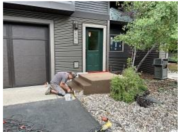
Building C4 Unit 37 Stoop Coating Began
