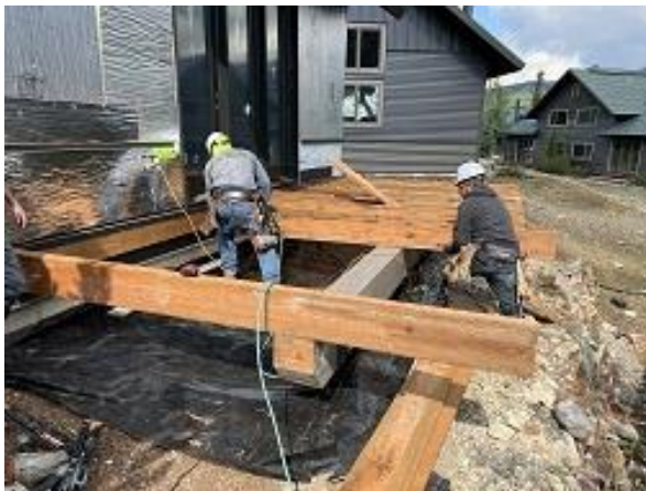
Building C10 Unit 69 Deck Framing
