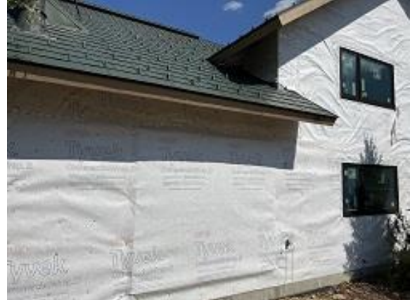
Building C4 Unit 35 Back Windows Installed
