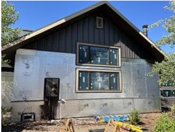
Building C10 Unit 70 Side Snap Batten Siding Installed
