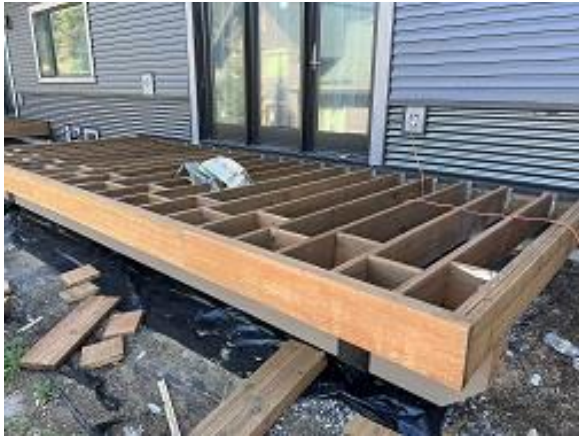
Building D Unit 37 Deck Framing
