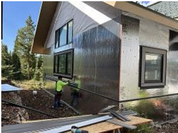
Building C6 Unit 54 Side Lap Siding Installed
