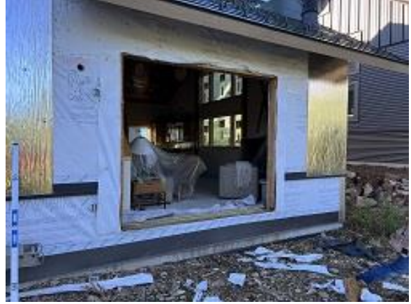
Building C6 Unit 54 Deck Door Removed
