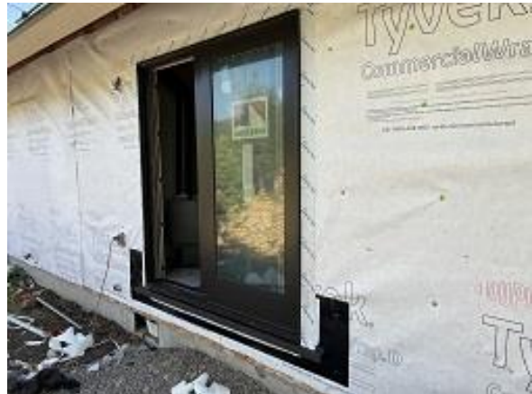
Building B Unit 4 Deck Door Installed
