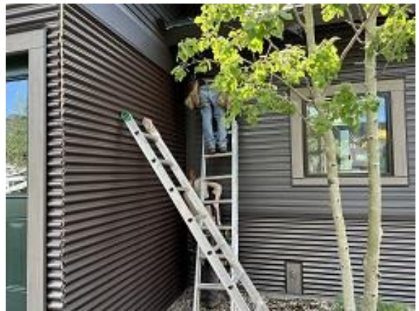
Building C7 Unit 59 Front Corners Installed
