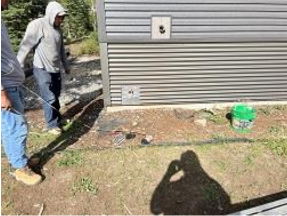
Building E8 Unit 58 Side Radon System Vent Blocking Location Cut
