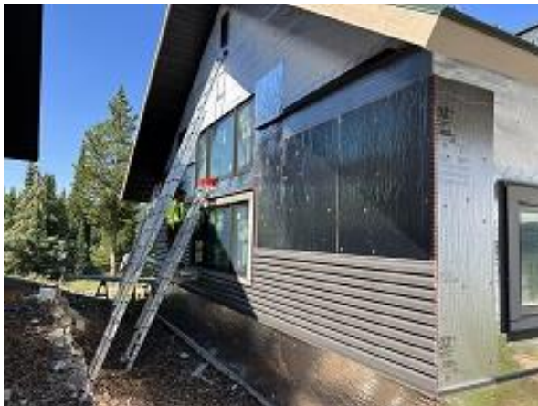
Building C6 Unit 54 Side Lap Siding Installed
