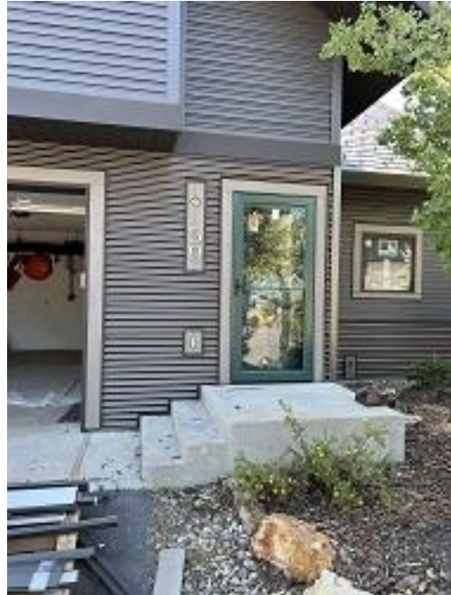
Building C7 Unit 59 Storm Door Installed
