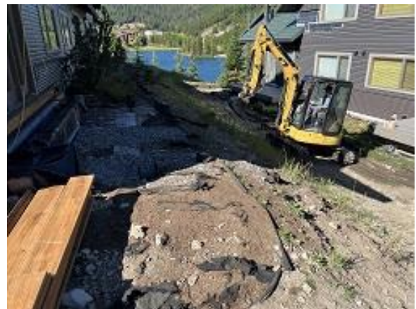
Building E5 Units 41 - 43 Required Clearance Grading Under Decks
