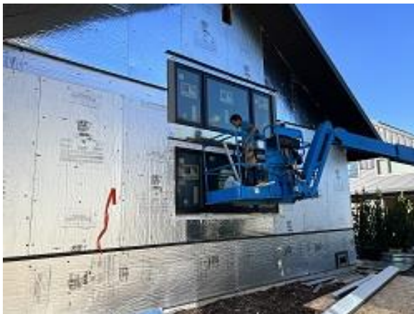
Building C10 Unit 69 Side Window Trim Installed
