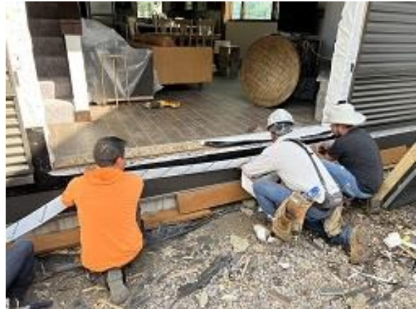
Building C5 Unit 39 Deck Door Flashing Tape Installed
