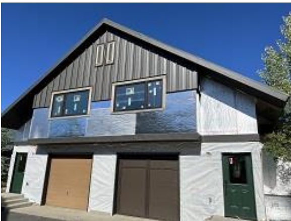
Building C10 Units 69 & 70 Front Snap Batten Siding Installed
