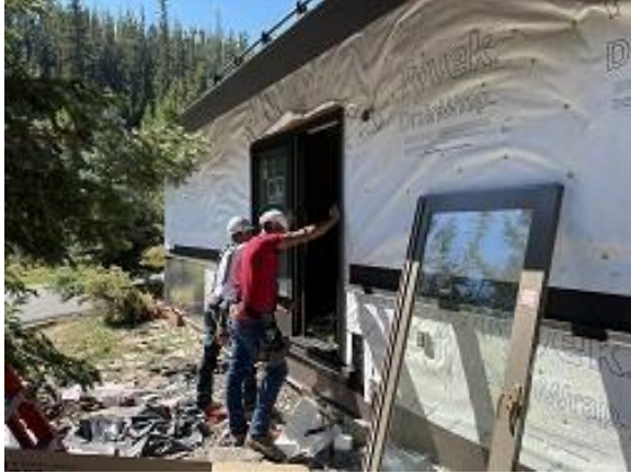
Building A Unit 1 Deck Door Installed
