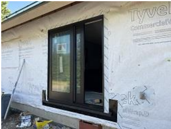
Building B Unit 3 Deck Door Installed
