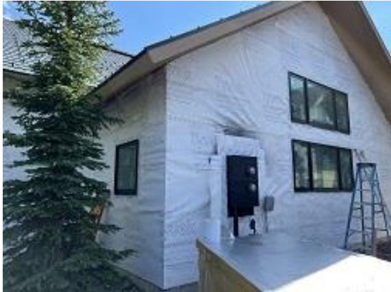
Building C4 Unit 35 Kitchen & Side Windows Installed
