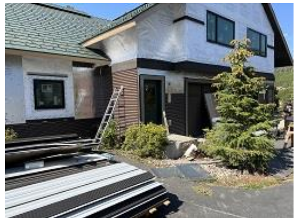
Building C6 Unit 54 Front Corrugated Siding Installed
