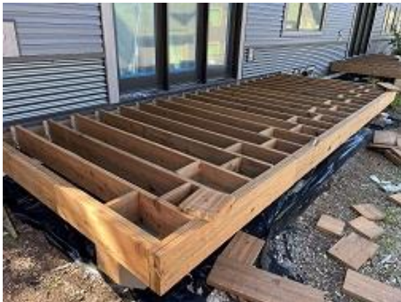
Building D Unit 36 Deck Framing
