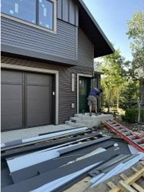
Building C7 Unit 59 Storm Door Installed
