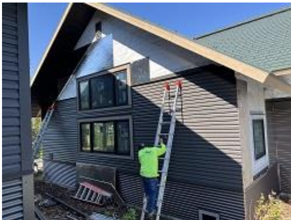
Building C6 Unit 54 Side Foam Board Insulation Installed
