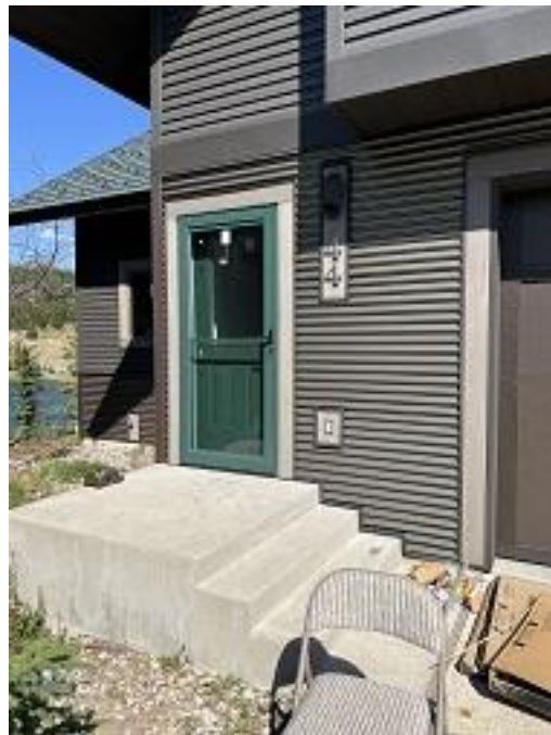
Building E5 Unit 44 Storm Door Installed
