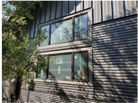
Building D Unit 36 Side Windows Installed
