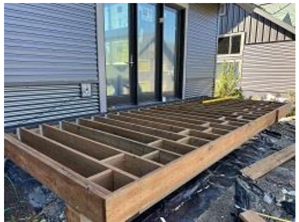
Building D Unit 38 Deck Framing
