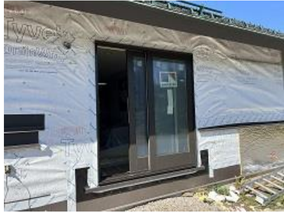
Building A Unit 2 Deck Door Installed
