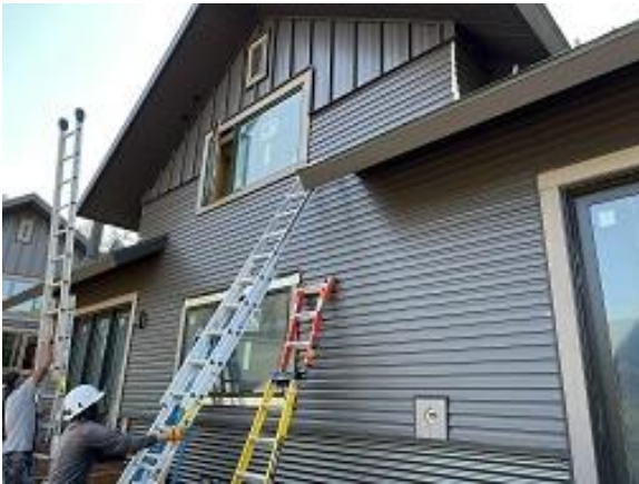
Building D Unit 36 Back Windows Installed
