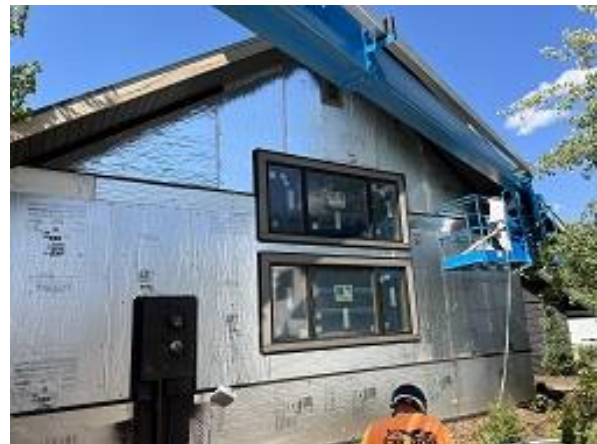
Building C6 Unit 53 Side Snap Batten J Channel Installed
