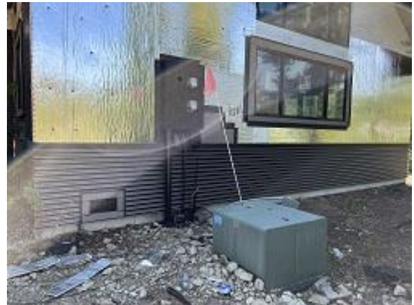
Building C6 Unit 53 Side Corrugated Siding Installed
