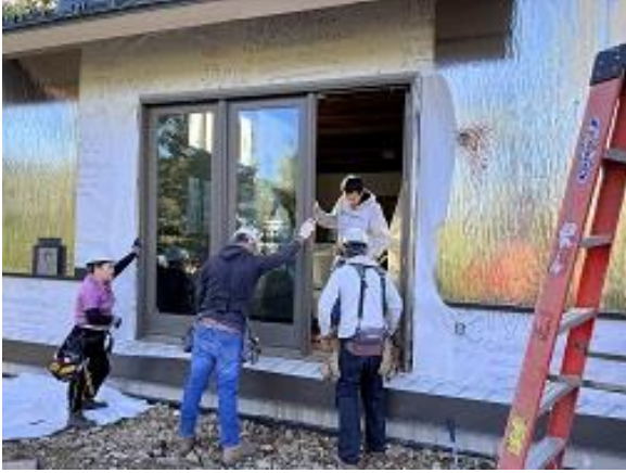
Building C6 Unit 53 Deck Door Removed
