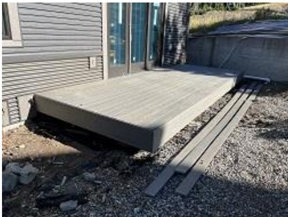
Building C9 Unit 68 Decking & Fascia Installed
