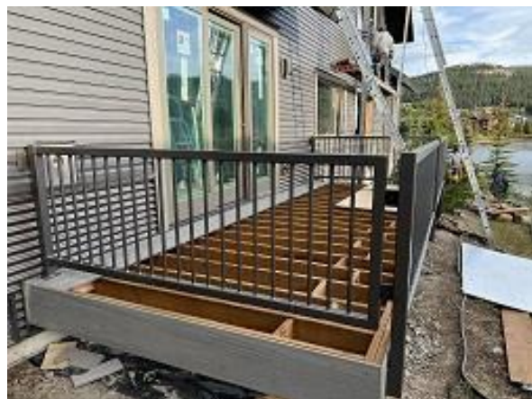
Building E5 Unit 43 Deck Railing Installed
