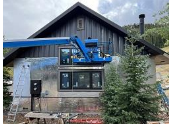
Building C4 Unit 35 Side Snap Batten Siding Installed
