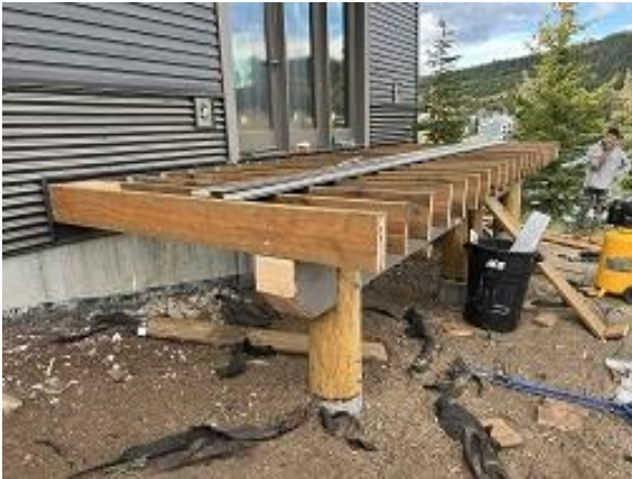
Building E5 Unit 44 Deck Joists Installed
