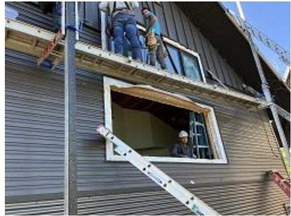
Building E5 Unit 44 Side Windows Installed
