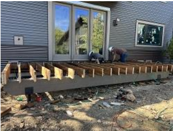
Building C10 Unit 70 Deck Framing Installed
