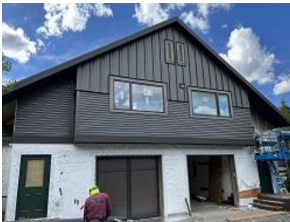
Building C4 Units 34 & 35 Front Lap Siding Installed
