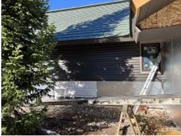
Building B Unit 4 Front Lap Siding Installed
