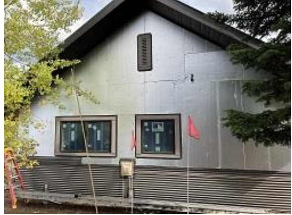
Building B Unit 7 Side Lap Siding Installed
