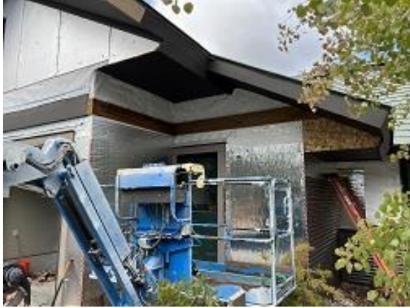
Building B Units 6 Front Belly Band Flashing Installed
