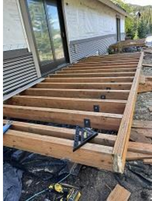
Building B Unit 6 Deck Framing
