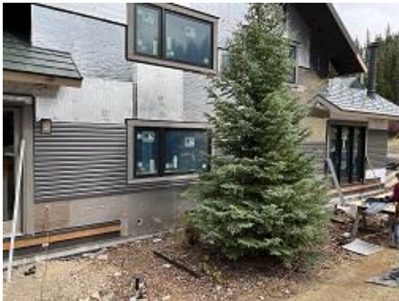
Building C4 Units 34 & 35 Back Lap Siding Installed
