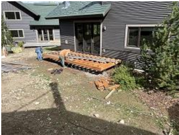
Building C5 Unit 40 Deck Framing Completed
