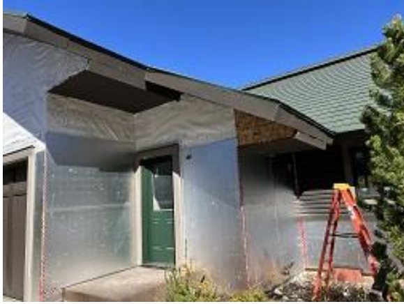
Building B Unit 3 Front Fascia Installed
