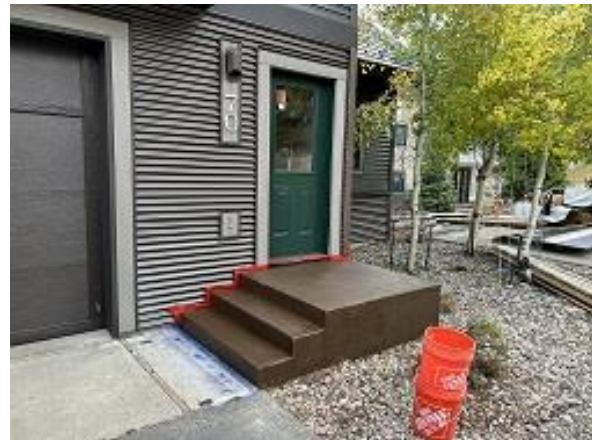
Building C10 Units 70 Stoop Refinishing Completed
