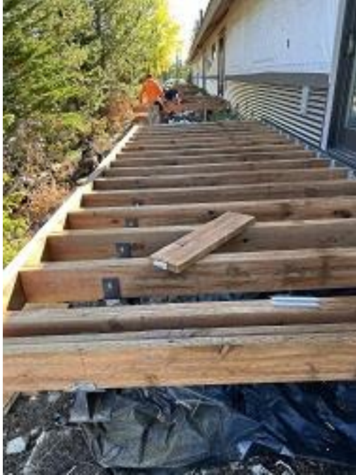
Building B Unit 7 Deck Framing
