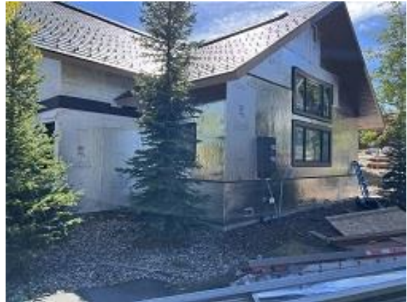
Building C4 Unit 35 Side Foam Insulation, Window Trim Installed
