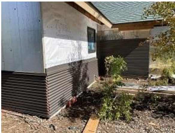
Building B Unit 7 Front Corrugated Siding Installed
