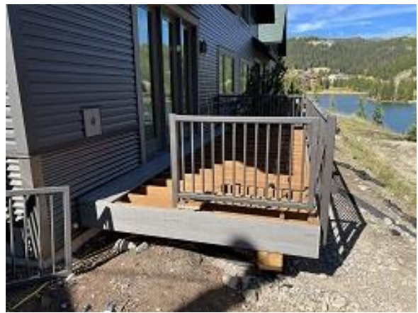
Building E5 Unit 41 Deck Railing Installed
