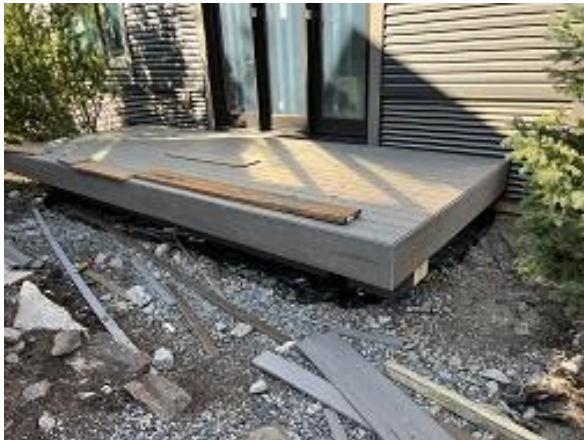
Building C2 Unit 14 Decking & Fascia Installed
