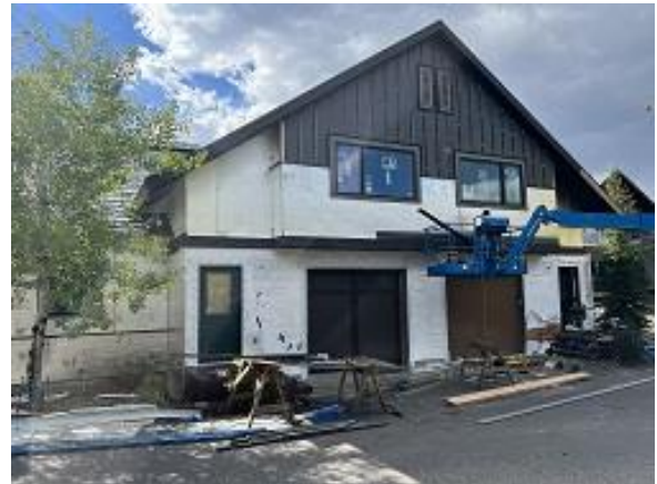
Building C4 Units 34 & 35 Front Snap Batten Siding Installed
