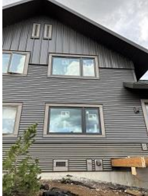
Building E5 Unit 44 Back Windows Installed
