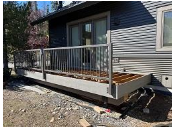
Building C3 Unit 32 Deck Railing Installed
