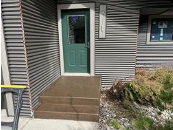
Building A Unit 1 Stoop Refinished
