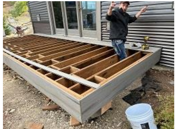
Building C10 Unit 70 Deck Fascia Installed
