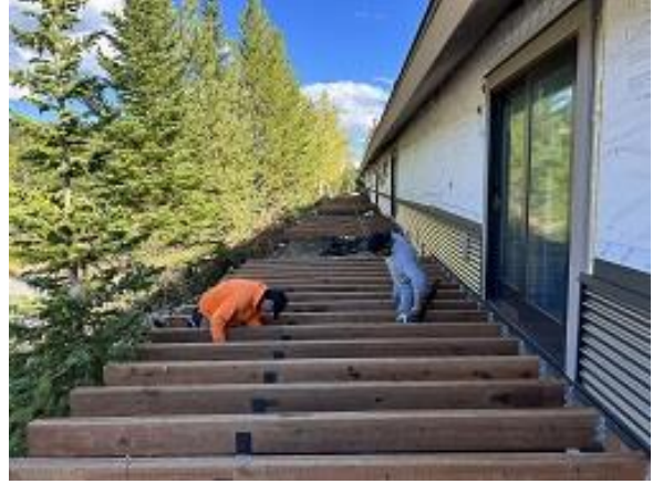
Building B Units 3 - 7 Deck Joists Install Continued
