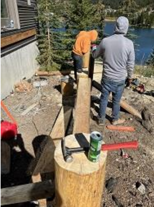
Building E5 Unit 44 Deck Framing Continued
