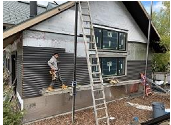
Building C4 Unit 34 Side Lap Siding Installed
