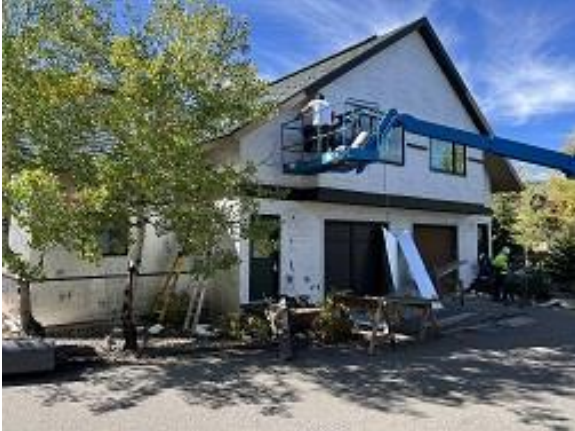
Building C4 Units 34 & 35 Front Belly Band & Snap Batten Flashing Installed
