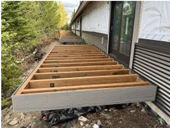
Building B Unit 7 Deck Fascia Installed
