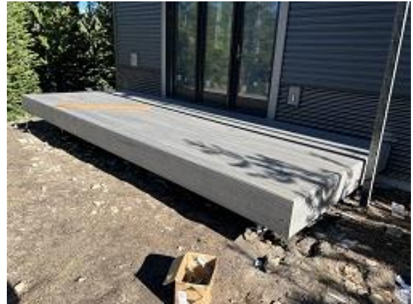
Building C6 Unit 53 Decking & Fascia Installed
