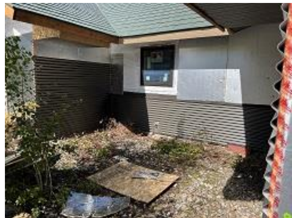
Building B Unit 6 Front Corrugated Siding Installed
