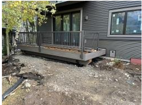
Building C1 Unit 12 Deck Railing Installed
