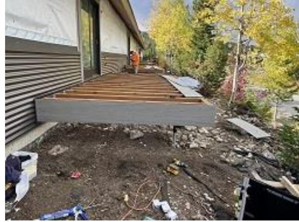
Building B Unit 3 Deck Fascia Installed
