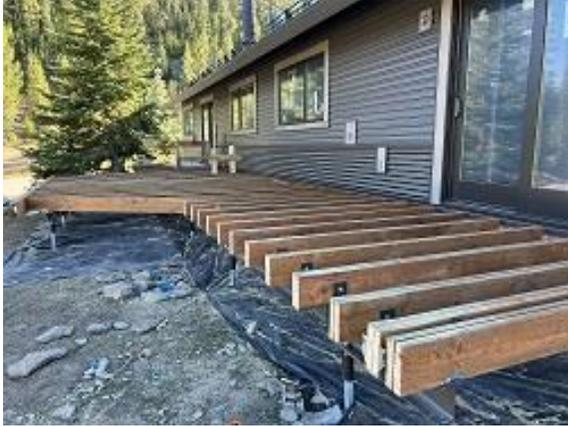
**Building A Units 1 & 2 Deck Framing & Lap Siding Installed**
