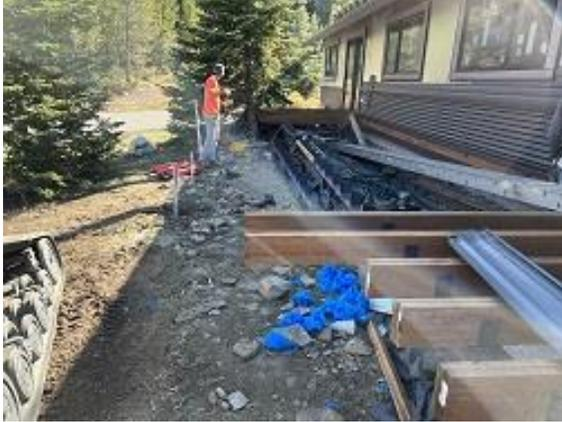
**Building A Units 1 & 2 Deck Helical Piers Relocated & Back Lap Siding Installation Began**
