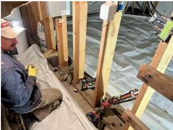
**Building C4 Unit 35 Crawl Space Radon Vapor Barrier**
