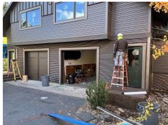
**Building C4 Units 34 & 35 Front Diverters, Corrugated & Lap Siding Installed**
