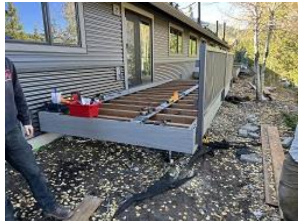
Building B Unit 4 Deck Railing Installed
