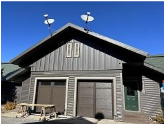
Building B Units 3 & 4 Satellite Dish Installed
