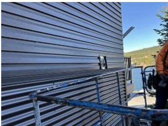
Building F1 Unit 16 Side Fireplace Vent Blocking Installed
