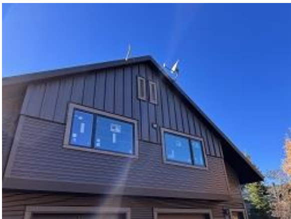
Building C4 Units 34 & 35 Satellite Dishes Installed
