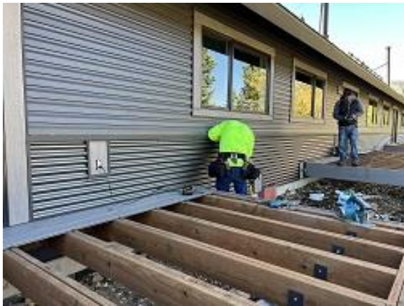
Building B Units 3 & 4 Back Corrugated Siding Installed
