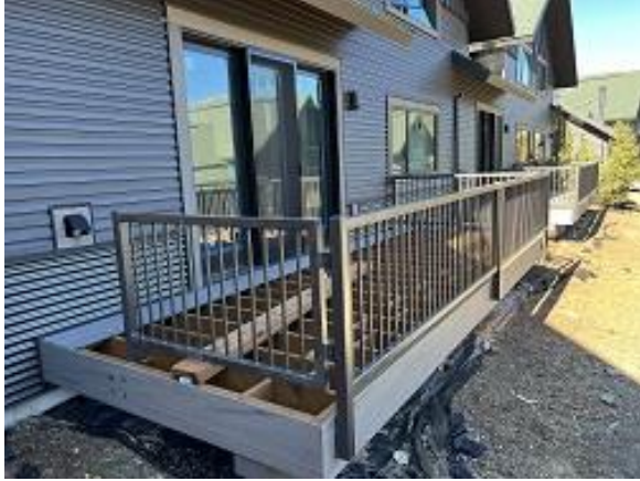
Building D Unit 36 Deck Railing Installed
