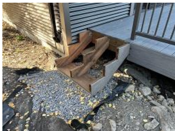
Building D Unit 36 Deck Stairs Installed
