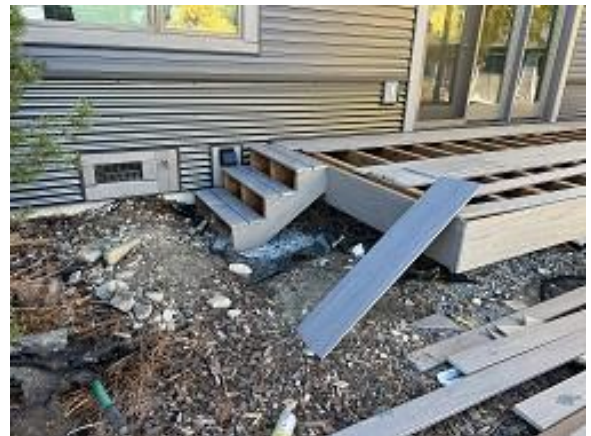
Building E9 Unit 61 Deck Steps Installed
