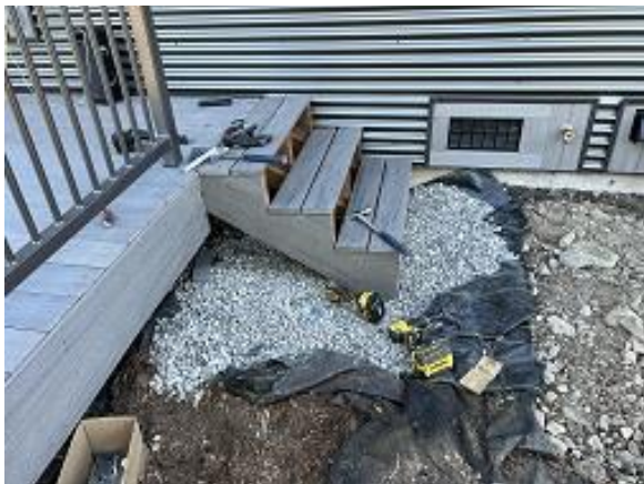
Building E8 Unit 57 Deck Steps Installed
