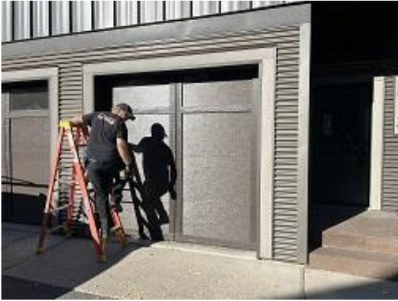
Building B Unit 3 Garage Weather Stripping Installed
