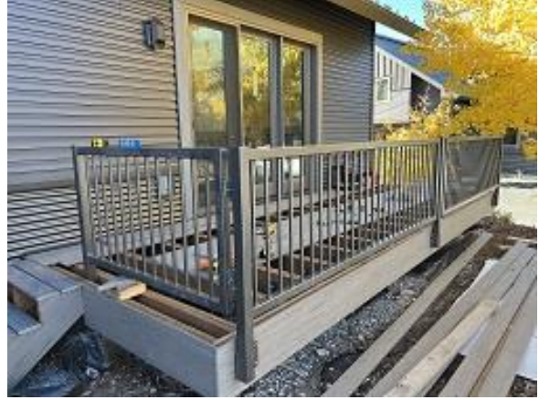
Building E9 Unit 61 Deck Railing Installed
