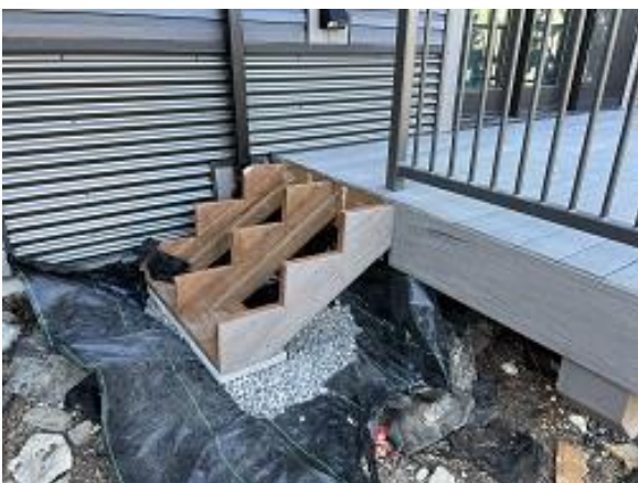
Building D Unit 37 Deck Stairs Installed
