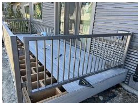
Building E5 Unit 42 Decking Installed
