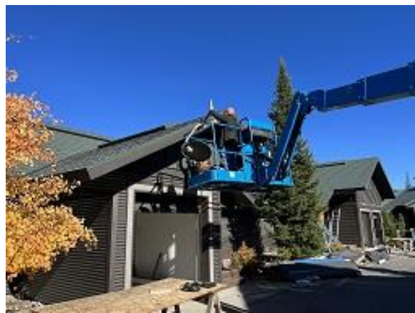
Building B Unit 5 Satellite Dish Installed
