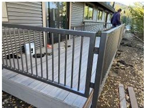
Building B Unit 5 Decking Installed
