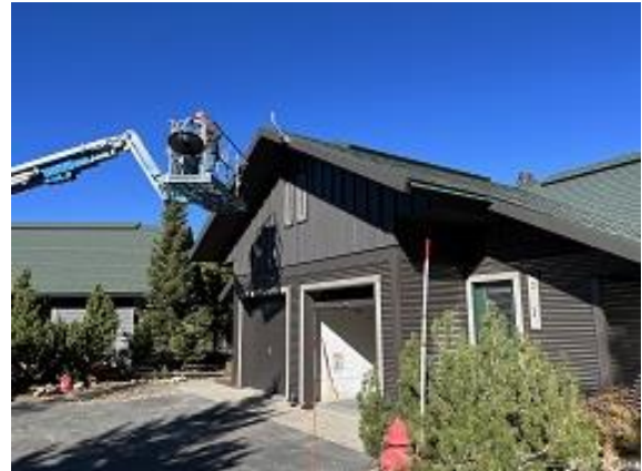
Building A Units 1 & 2 Satellite Dish Installed
