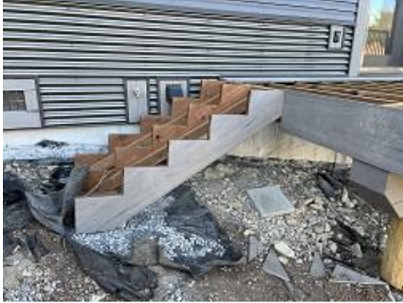
Building E5 Unit 44 Deck Stairs Installed
