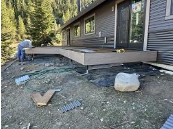
Building A Unit 2 Deck Fascia Installed
