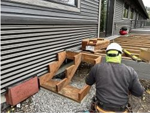
Building B Unit 3 Deck Stairs Installed
