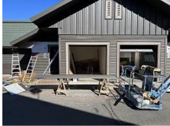
Building B Units 3 & 4 Front Corrugated Siding Installed
