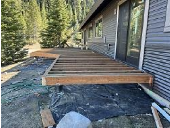
Building A Units 1 & 2 Deck Framing Completed
