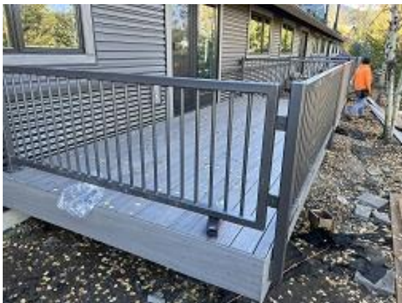
Building B Unit 4 Decking Installed
