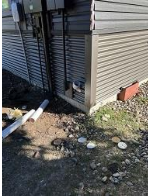
Building A Units 1 & 2 Radon Exhaust Installed
