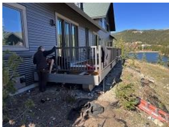
Building E5 Unit 42 Deck Railing Installed
