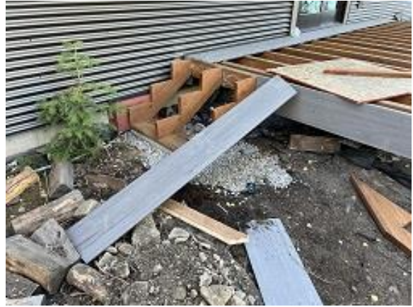
Building B Unit 6 Deck Stairs Installed
