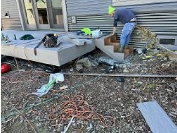
Building E9 Unit 64 Deck Stairs Installed
