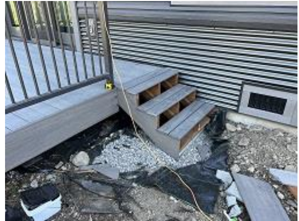
Building E8 Unit 55 Deck Steps Installed
