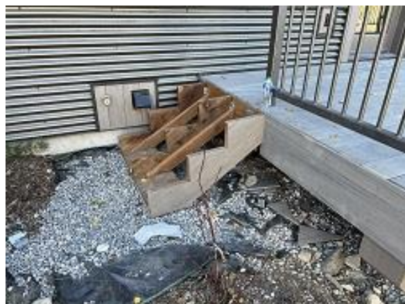
Building E9 Unit 42 Deck Stairs Installed
