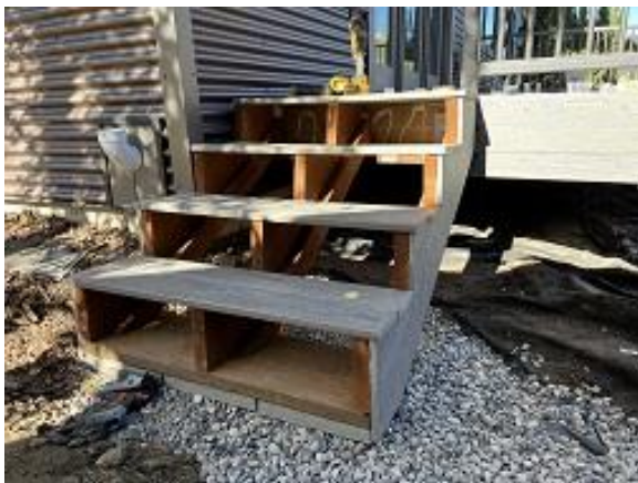
Building C10 Unit 70 Deck Stairs Installed
