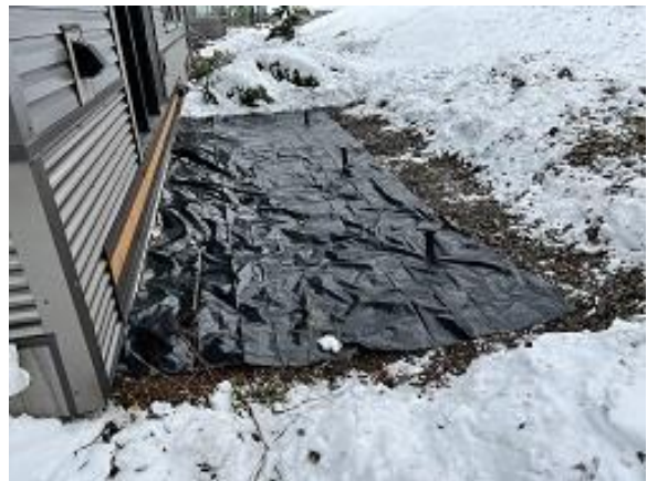
Building C8 Unit 65 Deck Plastic Installed
