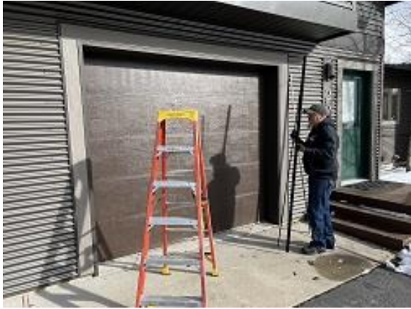
Building E3 Unit 25 Garage Door Weather Stripping Installed
