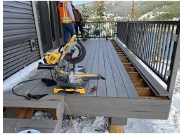
Building E5 Unit 44 Decking Installed
