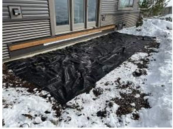
Building C9 Unit 67 Deck Plastic Installed
