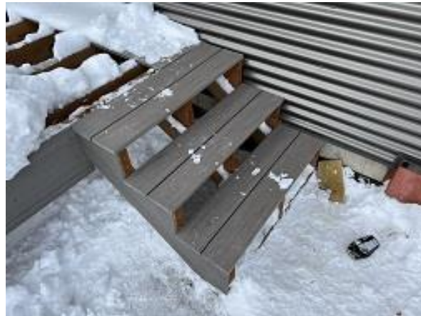
Building B Unit 7 Deck Stairs Installed
