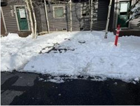
Building E3 Unit 25 & 26 Front Parking Area Materials Removed
