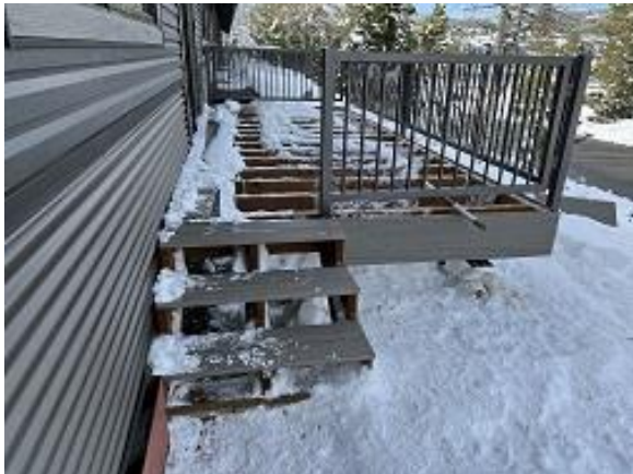
Building B Unit 3 Deck Railing Installed
