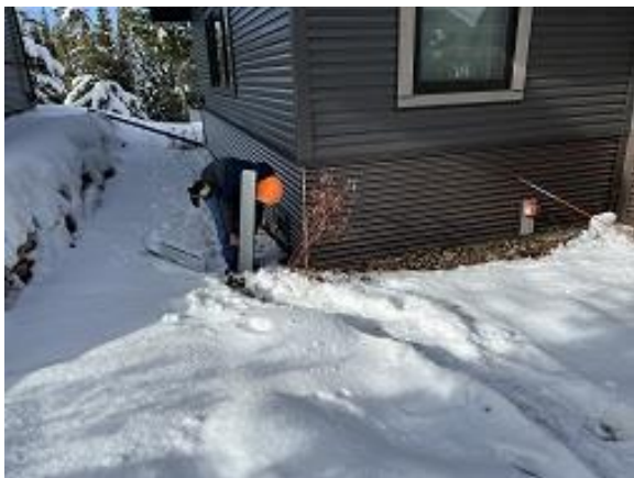
Building C6 Unit 54 Front Corner Installed
