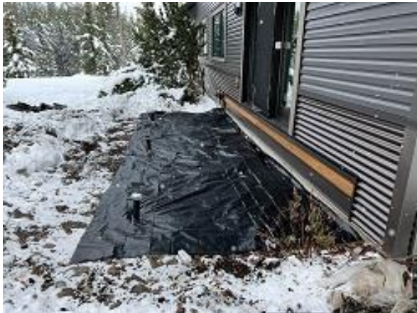
Building C7 Unit 60 Deck Plastic Installed
