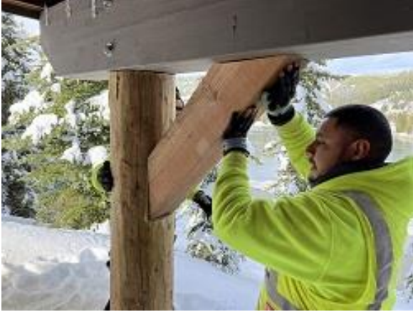
Building E7 Unit 52 Deck Knee Braces Installed
