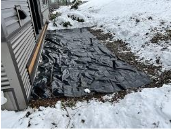
Building C8 Unit 65 Deck Plastic Installed
