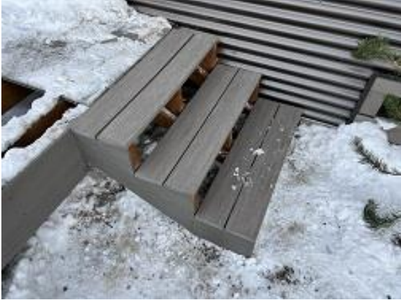
Building C6 Unit 53 Deck Stairs Installed
