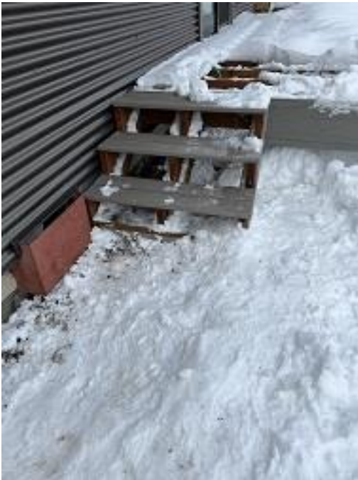
Building B Unit 3 Deck Stairs Installed
