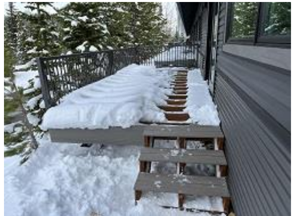
Building B Unit 7 Deck Railing Installed
