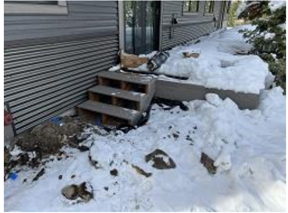
Building A Unit 1 Deck Railing Installed
