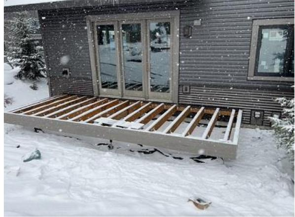
**Building C4 Unit 35 Side Deck Framing Completed & Fascia Installed**
