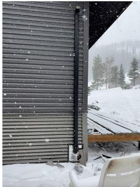
**Building C8 Unit 65 Side Radon Exhaust Installed**
