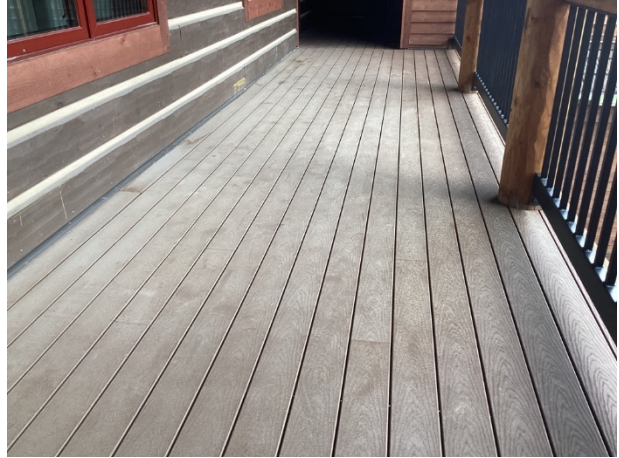
Composite breezeway deck at Building Two
