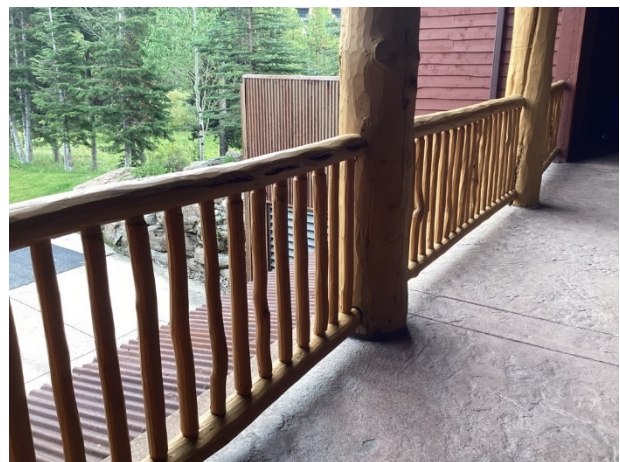
Wood railings at Building One
