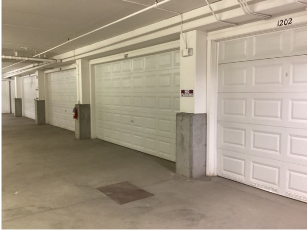
Unit owner garage doors
