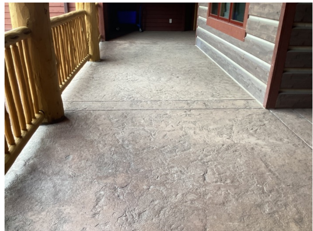
Concrete breezeway at Building One
