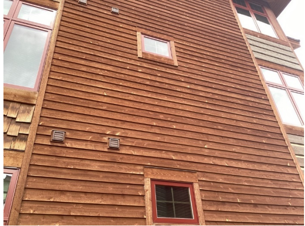
Lap style wood siding at Building Two
