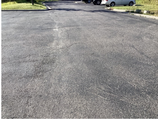
Asphalt pavement access drive overview
