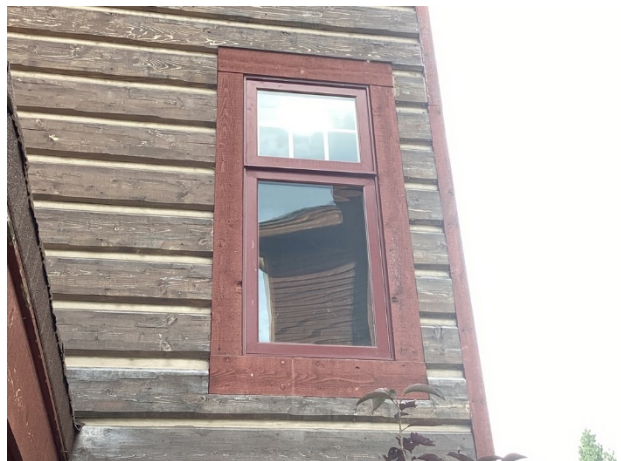
Aluminum cladding at common window
