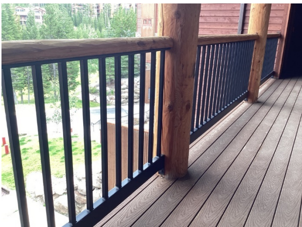
Steel railings at Building Two (Long lived)
