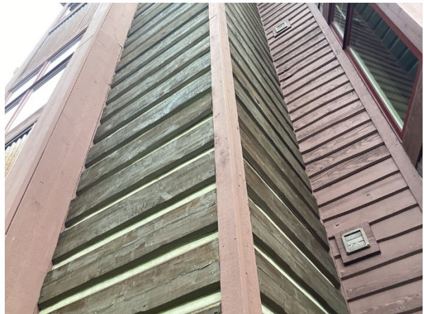
Log style siding at Building One
