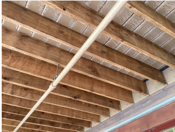
Breezeway wood frame
