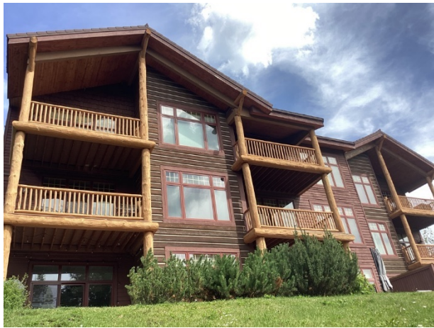
Building One exterior rear elevation view
