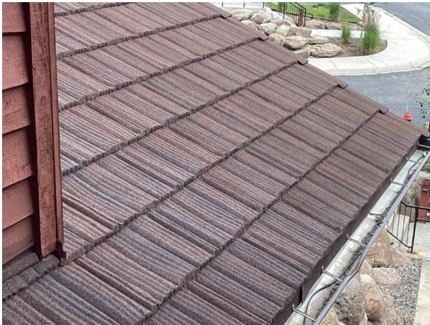
Stone coated metal roofing
