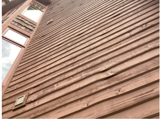
Lap wood siding at Building One
