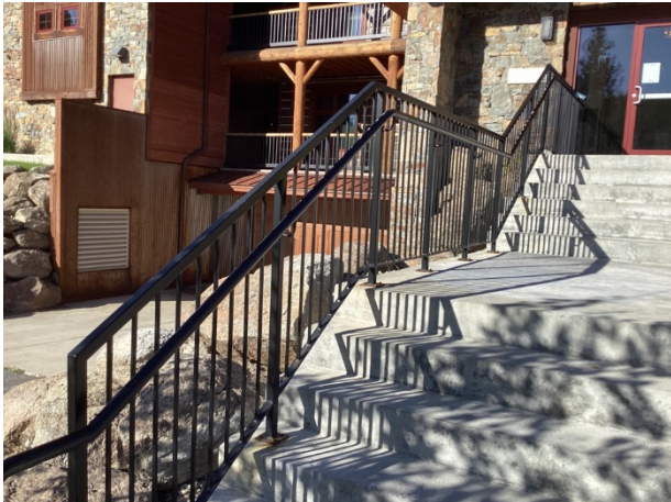
Building Two railing
