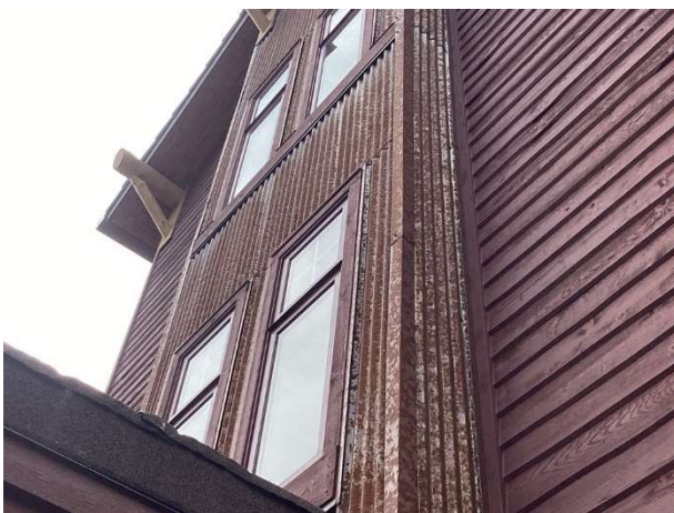
Walls, Steel Siding
