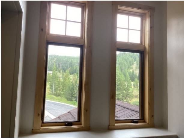
Common windows at stairwell
