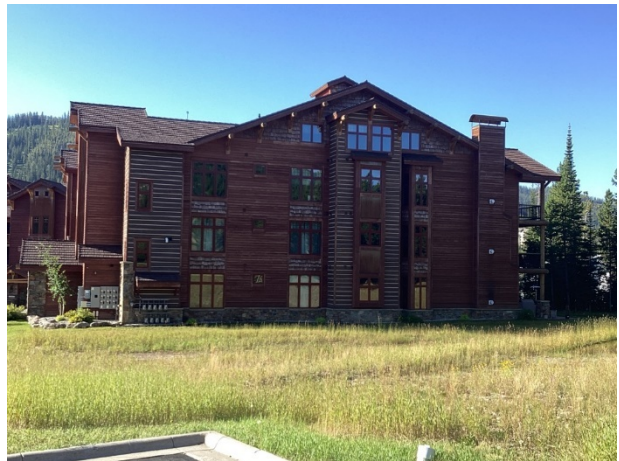
Building Two exterior side elevation view
