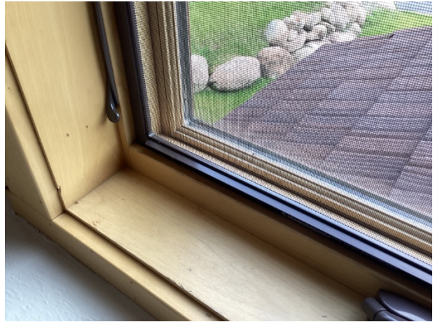
Wood frame windows
