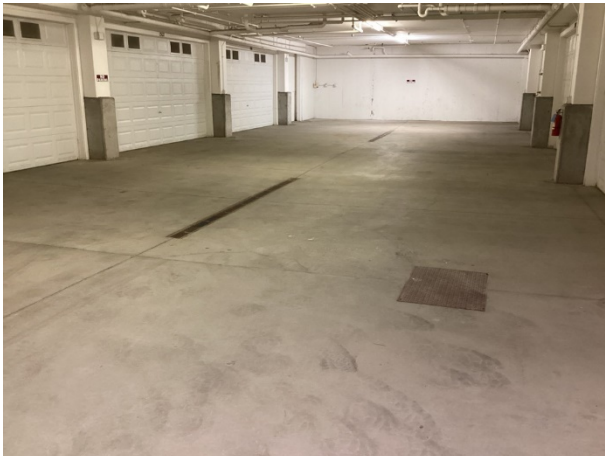
On-grade garage floor overview
