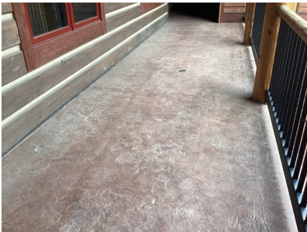
Concrete breezeway at Building Two
