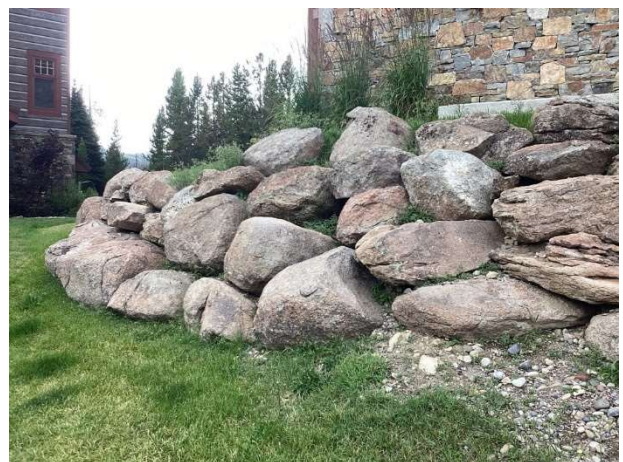
Stone boulder retaining wall
