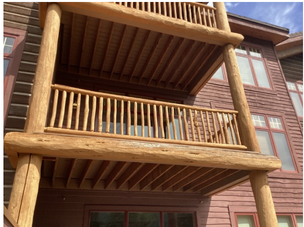
Unit balconies at Building One
