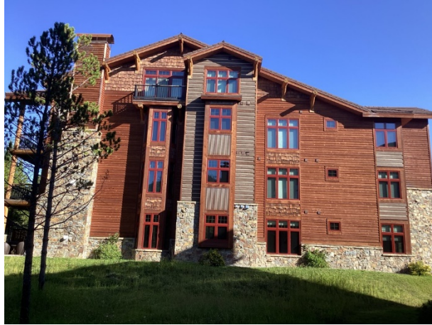
Building Two exterior side elevation view
