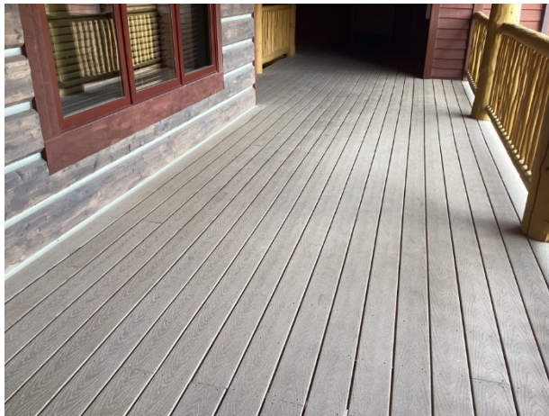
Composite breezeway deck at Building One
