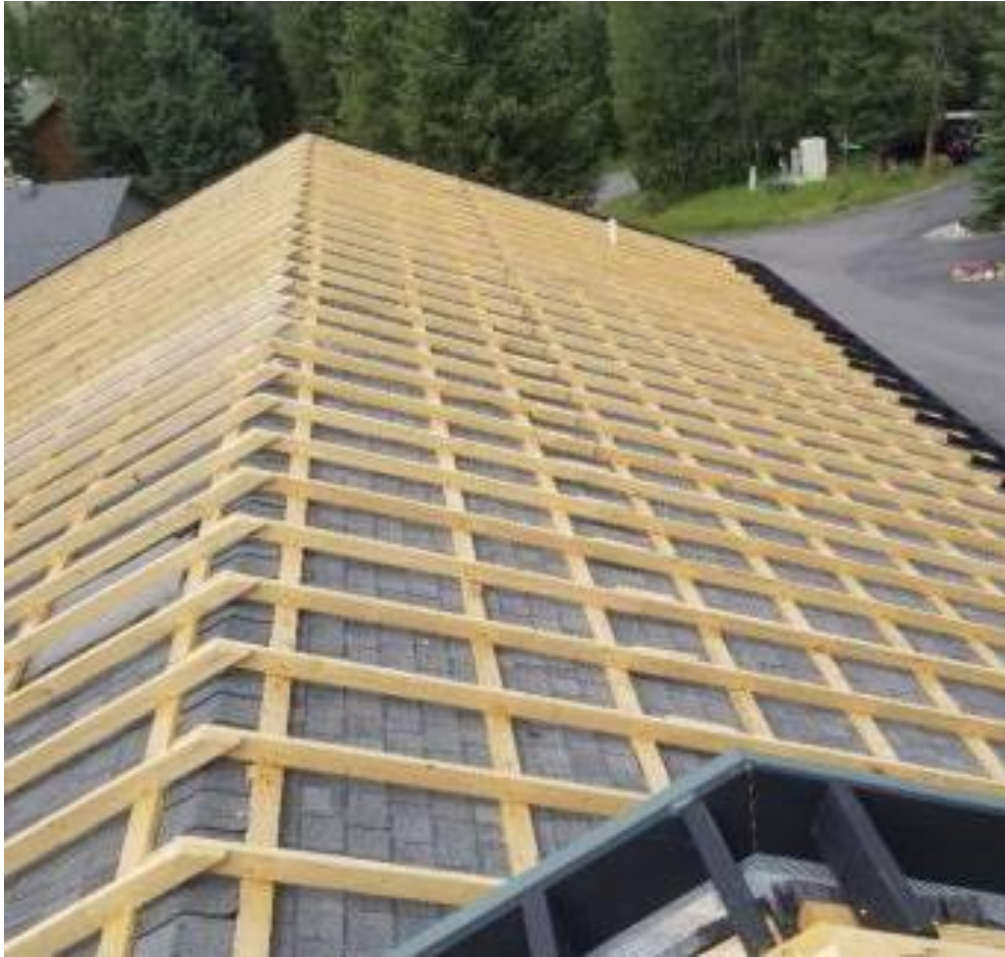
Cross framed cold roof buildout over existing
